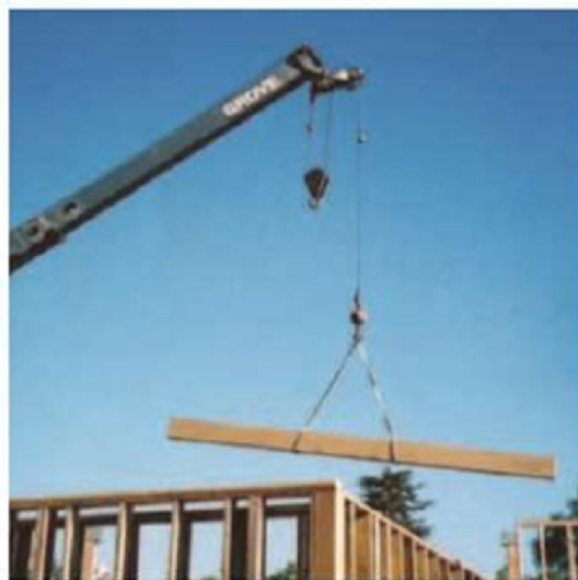
Overhead hazard – danger of falling material
